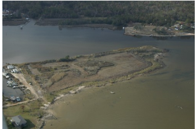
The newly graded and restored wetland, ready for planting.
