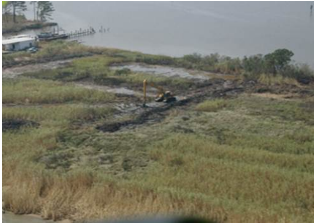
Tidal channels were reestablished, invasive plants were removed, and the fill was re-graded.
