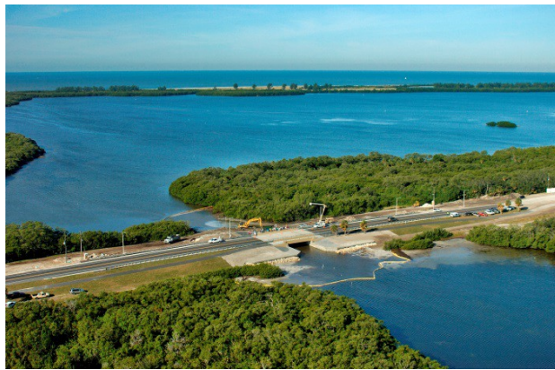
A causeway dike was replaced with a 40-foot span bridge.
