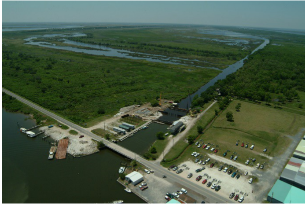
Construction begins on the water control structures.
